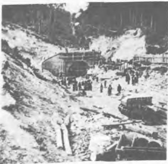
Construction of a railway tunnel in Paneriai near Vilnius (1861)
