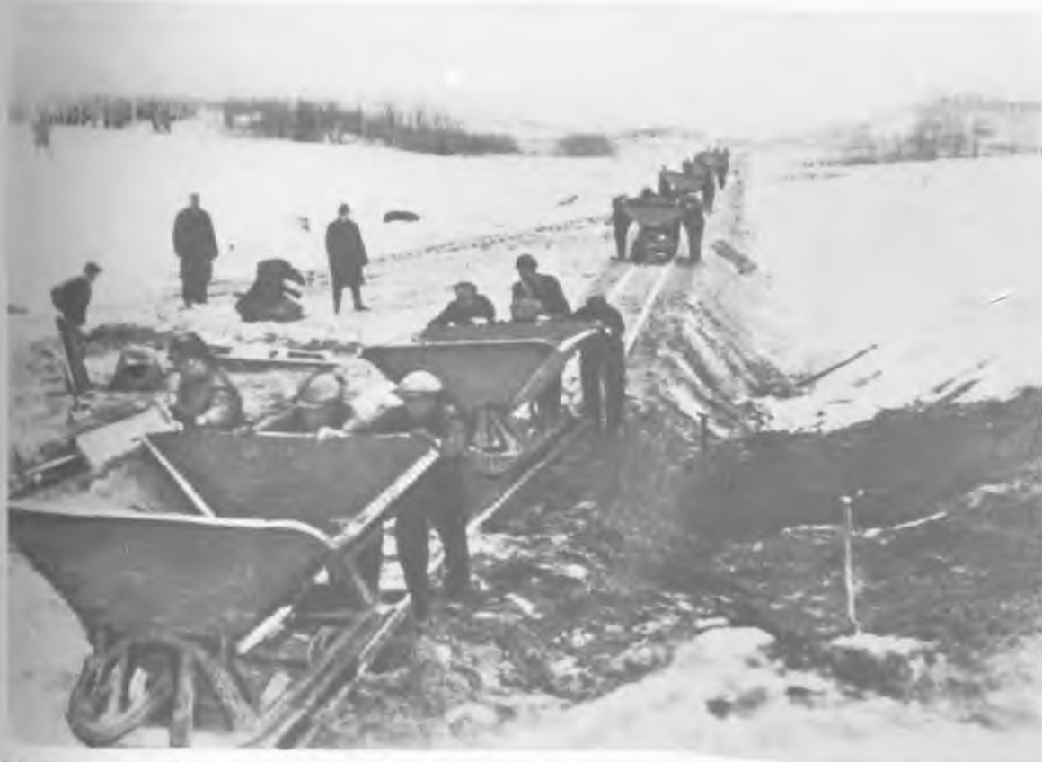
The 1930s: construction of the highway Kaunas—Klaipėda
